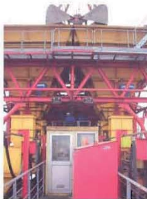
AIRCHOC at the CCI harbour in Calais (France).
