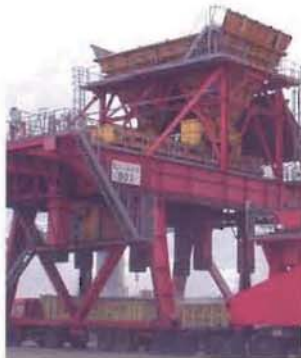
AIRCHOC at the CCI harbour in Calais (France).
